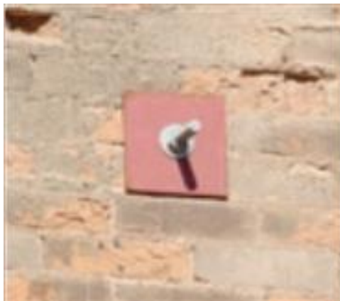
A steel plate with anchor bolts.
