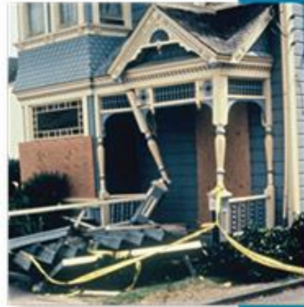
This older home collapsed after earthquake shaking damaged its crawl space (cripple) walls.
